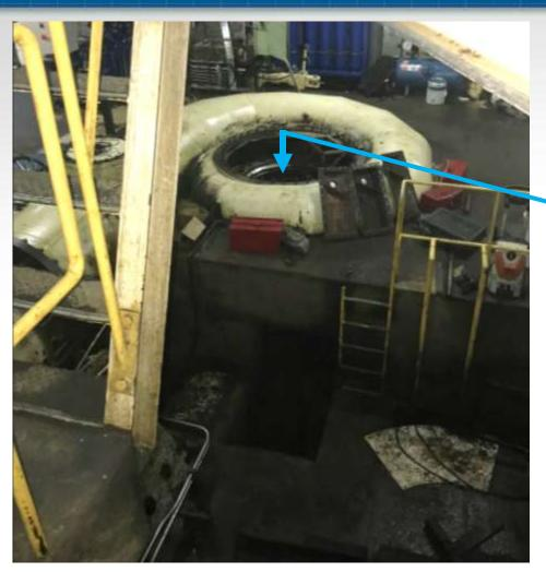
The Draft Tube is located over 200 Metres below Ground level and is inside this Pump Turbine
